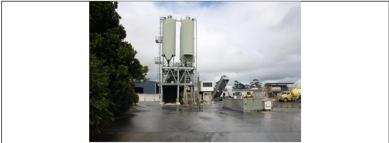
Figure 2: Hymix - Chinderah Concrete Plant
