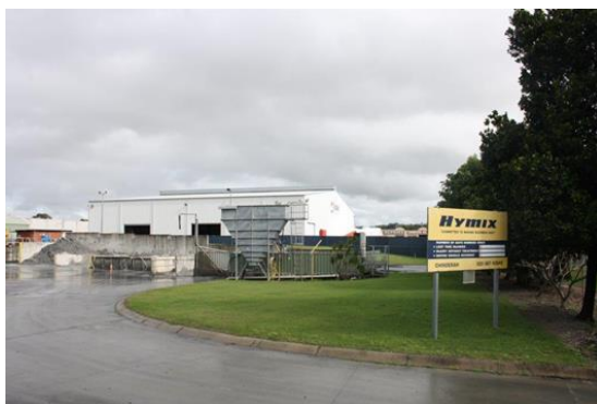
Figure 1: Hymix - Chinderah Concrete Plant
