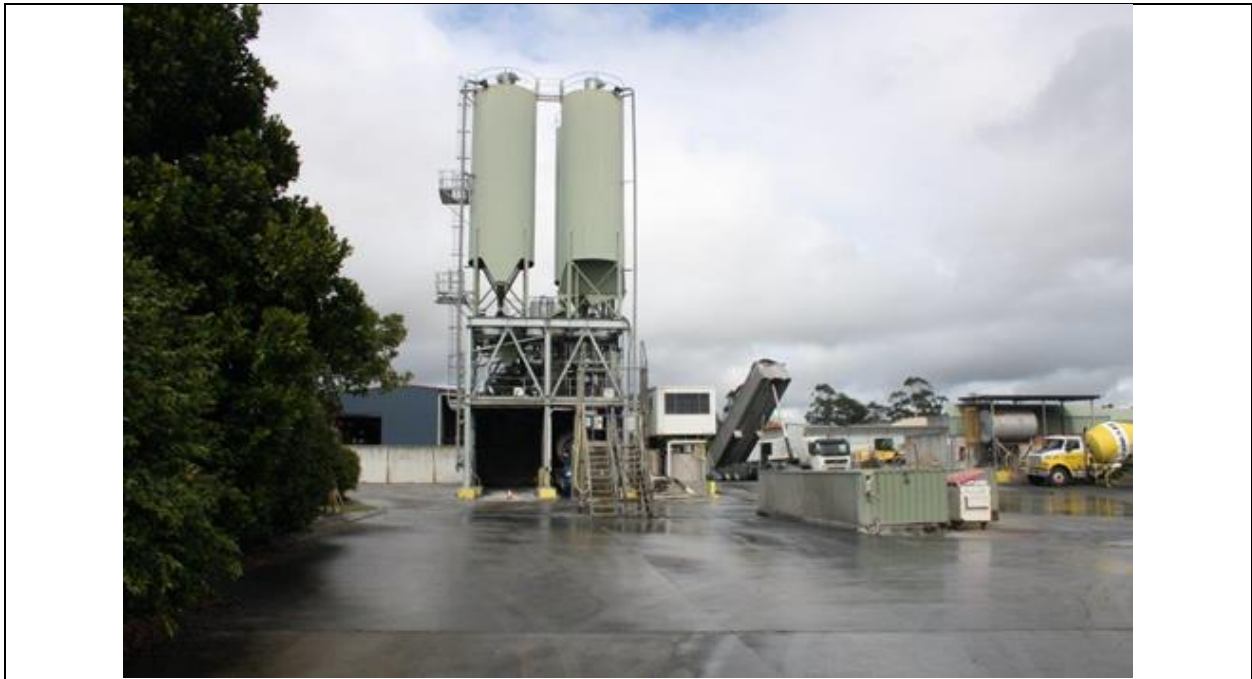
Figure 1: Hymix - Chinderah Concrete Plant
